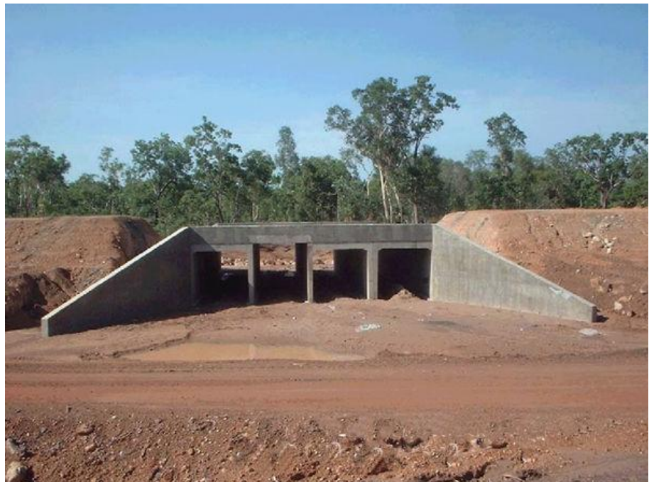
Figure 3-1 Concrete Box Culverts Under Railway (Source: Australasia Railway Corporation)
